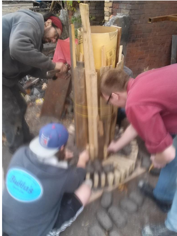
FIGURE 5. LAYERING CLAY ONTO FURNACE SIDES.
