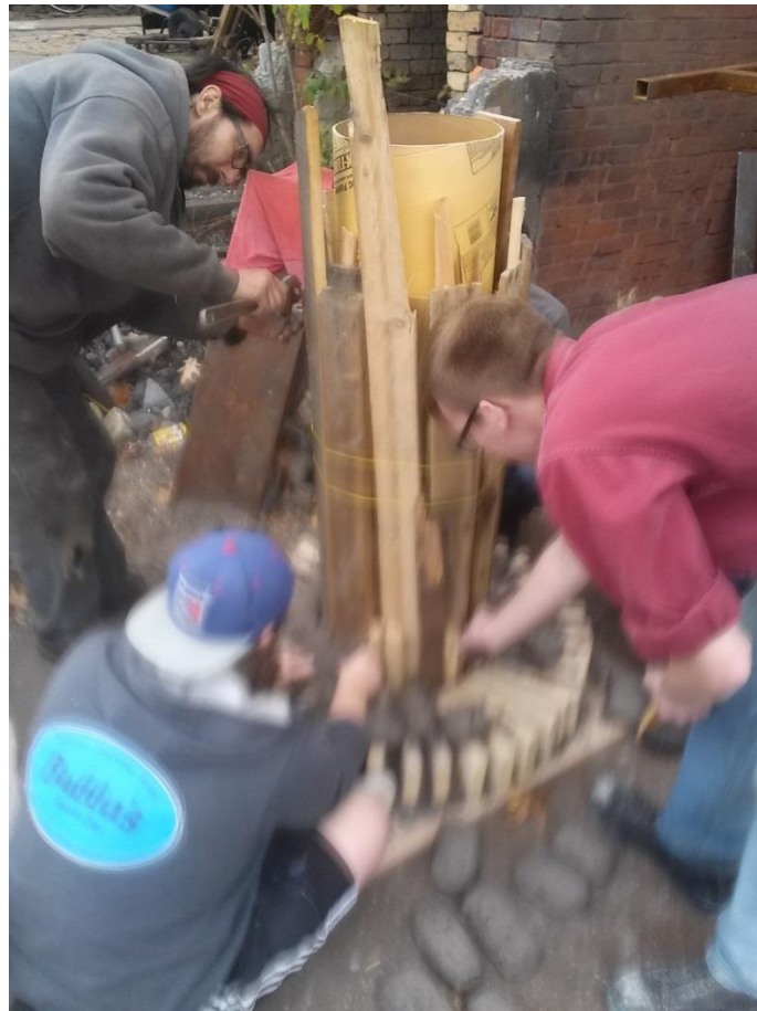
FIGURE 39. LAYERING CLAY ONTO FURNACE SIDES.
