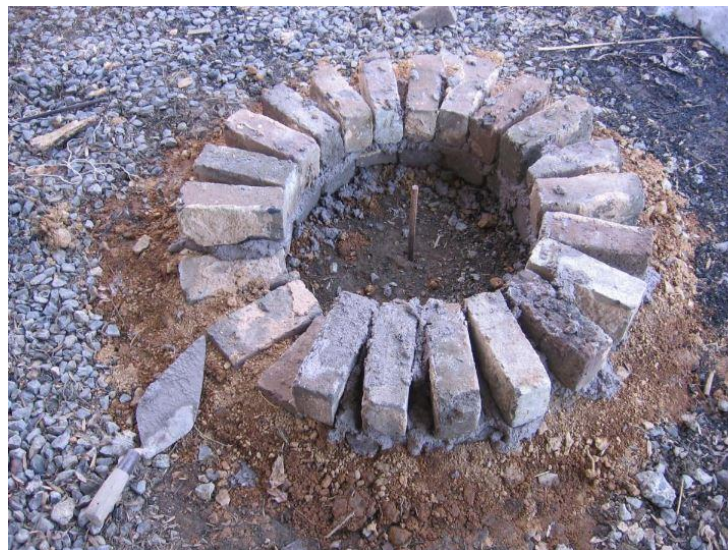
FIGURE 1. THE BASE OF THE FURNACE.
