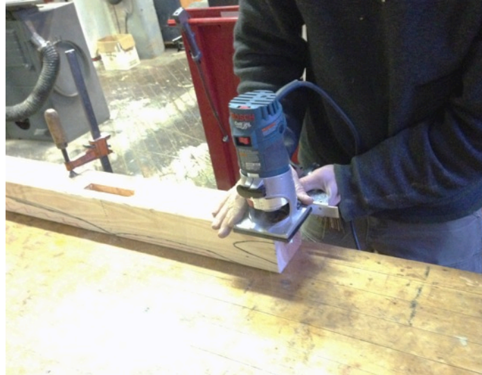
Figure 35: Making the canal for the bolt
