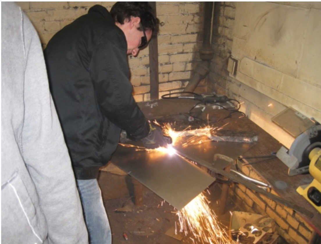
Figure 30: Using a plasma cutter to cut the sheet steel.
